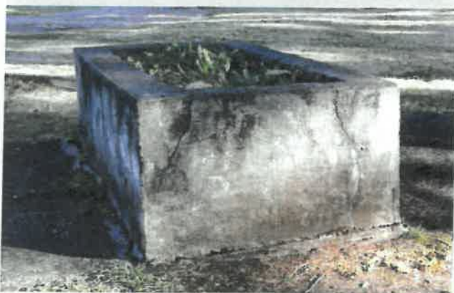
12. Concrete box near playground
