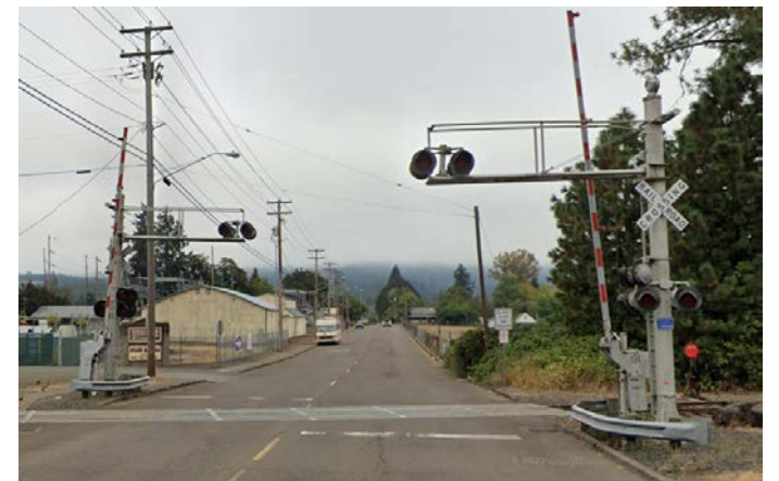
Figure 4: Rail crossing at 47th Avenue (Google Maps, 2022)
