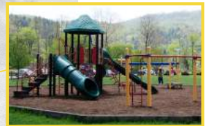
Existing playground equipment is clustered near parking and augmented with new elements
