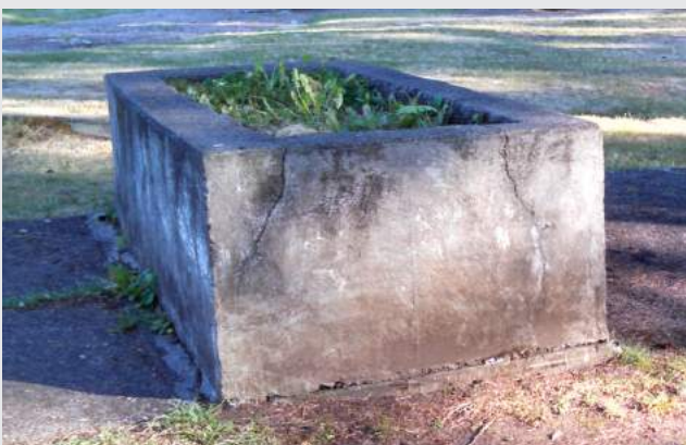
12. Concrete box near playground
