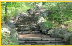
Stairs create a stronger connection between the Lower and Upper Sankey areas
